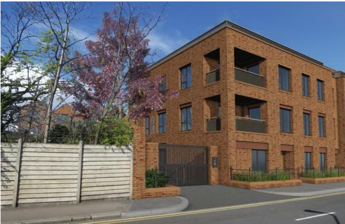
View from Hermitage Road (vehicular entrance)
